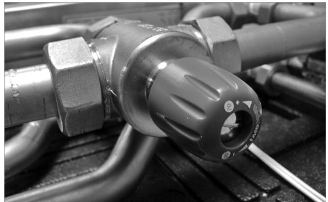
Fig. 25: Thermostatic mixing valve at WWS-36
