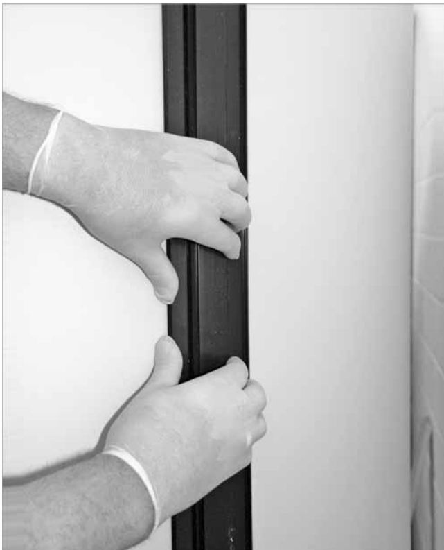
Fig. 7: Close the insulation sections
